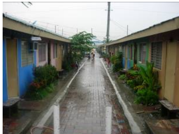
Housing for the urban poor – Gawad Kalinga, Manila
