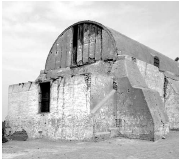
Pic. 8 Sacristy & head wall, 2005
