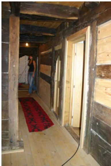
View of the hall in bedroom floor
