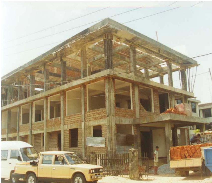
Fig 2: Super structure under progress
