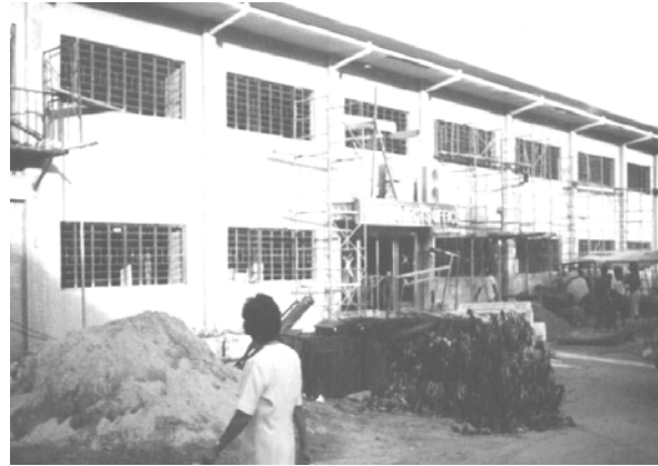
Figure 4. Construction in Progress
