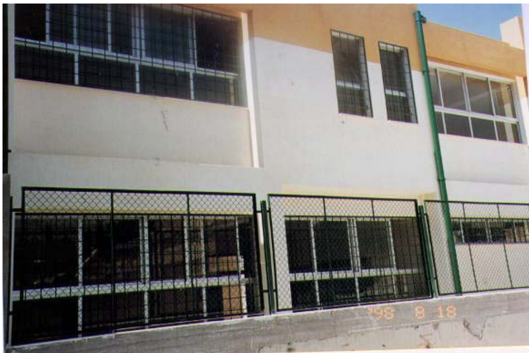
Photo 2: The Front Façade of Mazzeah School.
