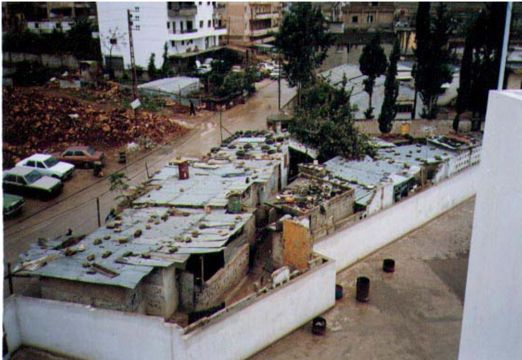
Photo 3 The site of the low cost housing project for displaced families at Beddawi Camp before construction – Lebanon
