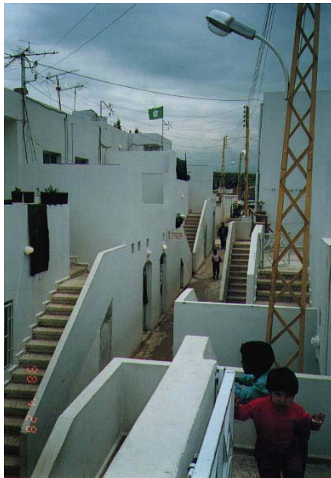
Photo 4 shows the entrance stair for a low cost housing project for displaced families at Beddawi Camp Lebanon.
