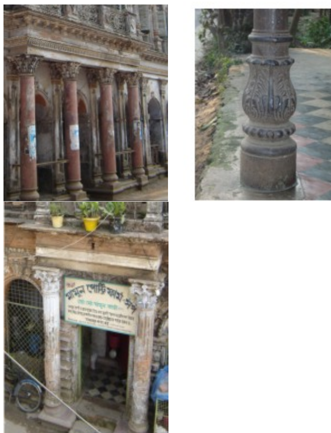
Fig. 10: Brick and iron columns placed on kalasa base and fluted column in the façade.
