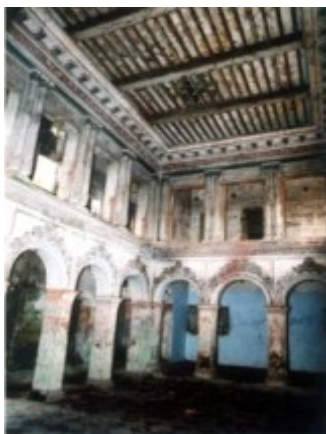
Fig. 02: (a) Plan of Central hall type Building no. 16 (b) View of a Central hall
