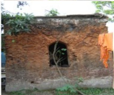
Fig. 05: Exterior View of Compartment type buildings number 41, 42 and 44 respectively.
