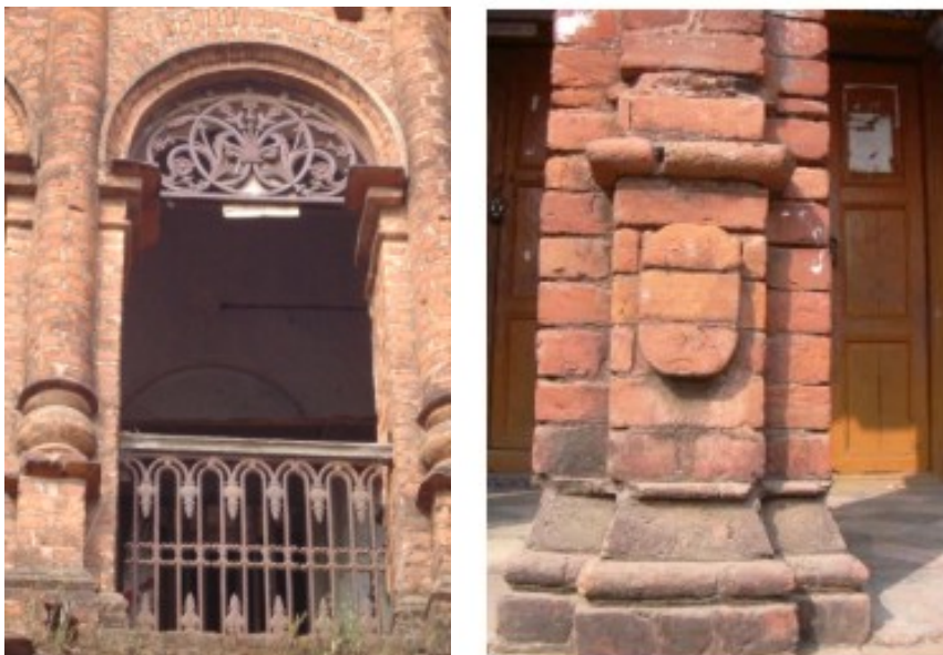
Fig. 11: Round and rectangular brick columns on moulding base in the buildings of Panam Street.
