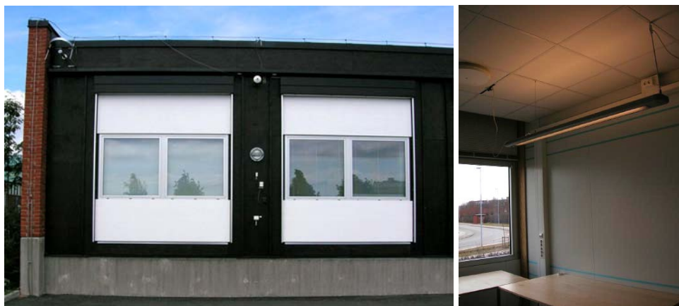
Figure 3.2 Exterior and interior of test room. The light sensor for controlling the venetian blind was placed on the facade between the rooms. The more open part of the venetian blind can be seen as a darker strip at the top of the windows in the room on the right.
