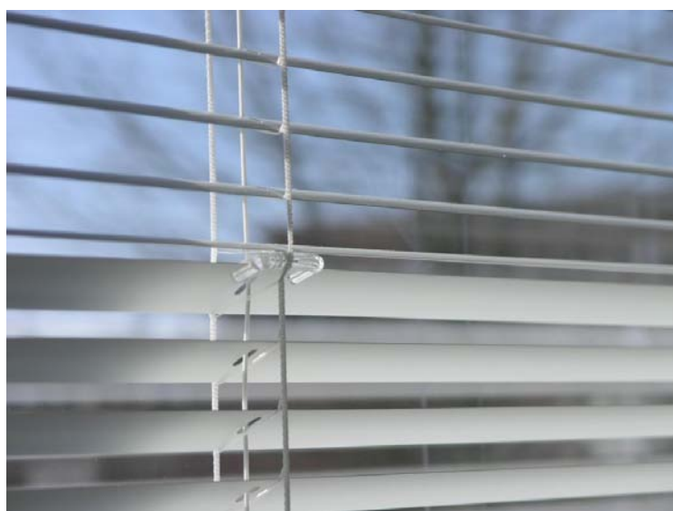
Figure 3.1 Picture of venetian blind with light redirection using clips. (Photograph: Thore Sonesson).
