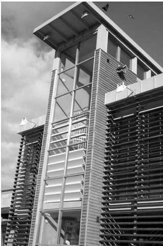
Figure 3: Illustration of integration of the Solar Window into the glazed façade of a staircase of an ecological exhibition building in Malmö.
