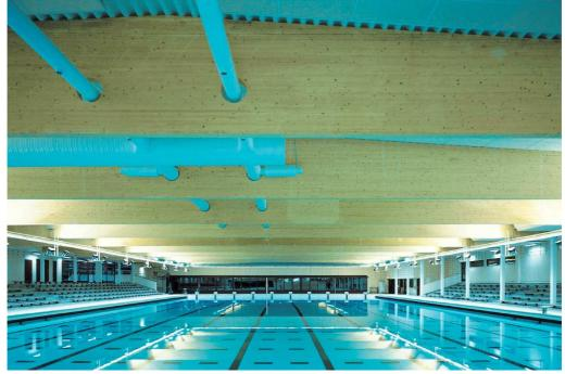
Figure 1.1: Examples of constructions with glulam beams with holes. Top: Restaurant Ideon, Lund, Sweden. Bottom: Indoor swimming pool, Västerås, Sweden (with permission from Martinsons Trä AB).
