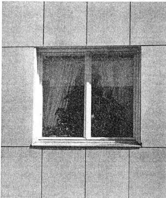
Above and below: Fig. 3 and 4. Part of façade before and after cladding. As also can be seen from fig. 7, detail 10, the fresh air inlets are covered. The fresh air is taken from the air space behind the cladding
