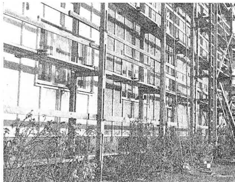
Fig. 6. Cladding of façade
