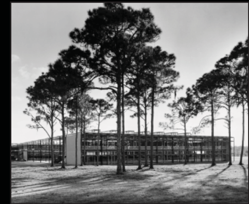
Riverview High School (1958) in Sarasota, Florida is a seminal post-World War II school designed by renowned architect Paul Rudolph.
